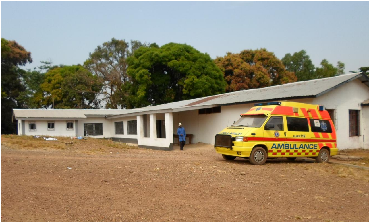
The east side of the unit and possibly the ambulance entrance in the future
